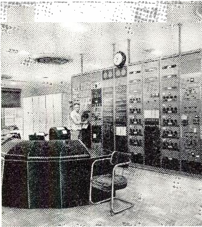
↑ Shown here is the main control console in the foreground. In the background may be seen the frequency shift exciters, the patch system, and the frequency counting equipment that is required at the communication center.
